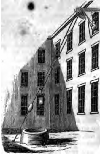
No. 15. Italian mode of raising water to the upper floors of a house.
